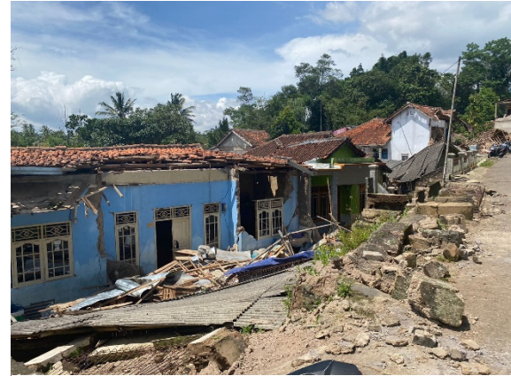
Damage to homes in Cianjur, Indonesia following the earthquake on November 21. Photo by Iswar Abidin for Project HOPE, 2022.
