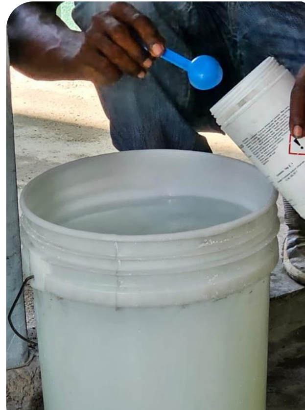
Water being disinfected through chlorination at a Project HOPE Cholera Treatment Center in Les Cayes, Haiti. Photo by Project HOPE staff, May 2023.
