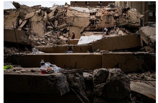
Collapsed residential buildings in Caracas. Photos: Ernesto Costante
